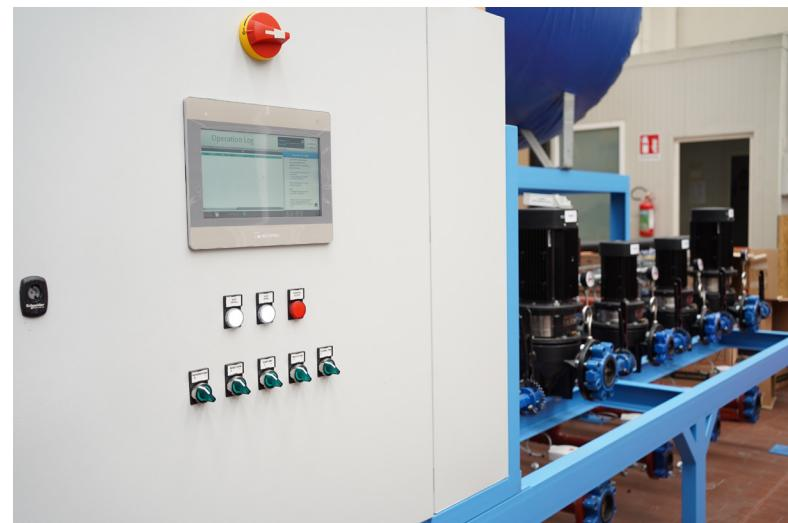
A mixer or blender for rubber and plastic production requires that a constant temperature be maintained in different sections of the plant. Picena Frigor designs and builds hydronic power plants with different utilities that can independently regulate the water temperature required for cooling. The hydronic power plant is in turn fed upstream by a chiller of adequate power, which is responsible for supplying the amount of chilled water required for subsequent regulation.
